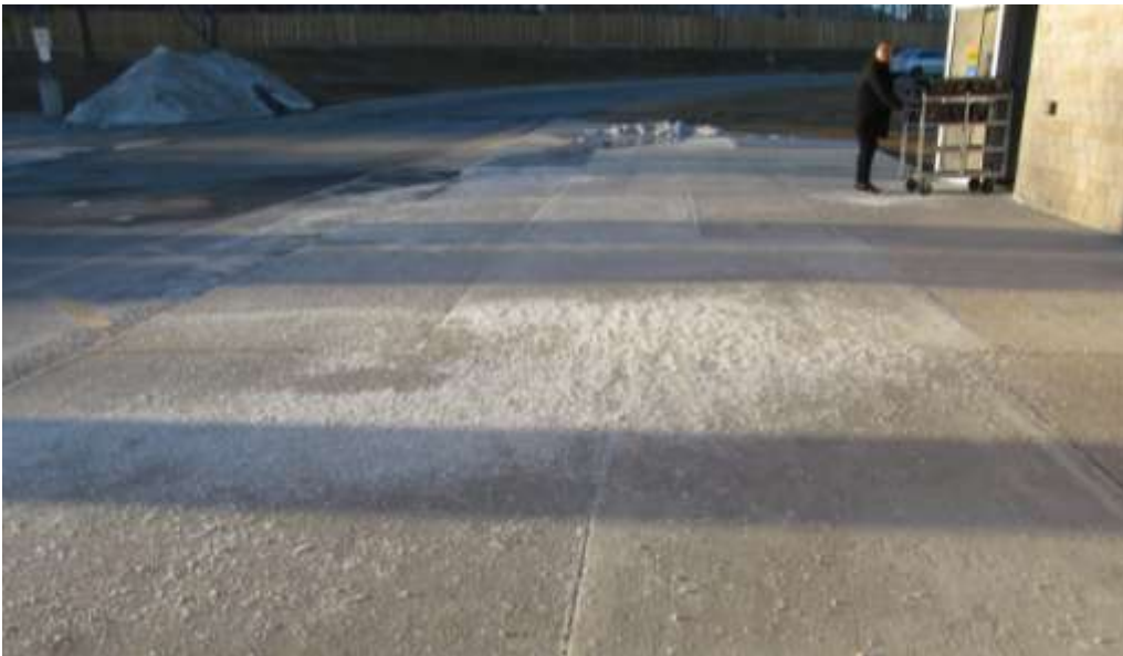
Over salting without calibrating equipment application in a grocery store area. (Lots of impervious pavement exacerbates the problem)
